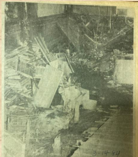
CLEAN UP CREWS were busy in the remains of Norm's Food Market Monday, and hope to finish the work by Friday, according to Norm Kibble. He said the news from Pierre, along with the fact that his wife, Dorothy, was scheduled to be released Tuesday from the hospital, should make it possible for him to make definite plans for the store soon. Leo Thomson, owner of Thompson's Clothing, which has been closed because of smoke damage, said Monday that he was waiting for action on USD/S and insurance before making future plans.
